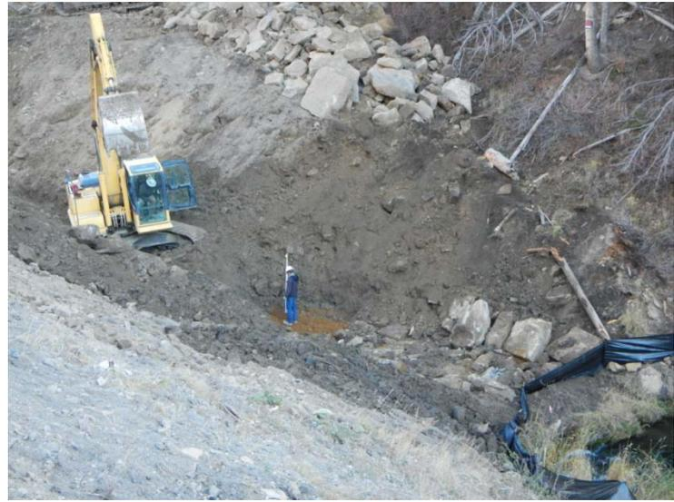
Checking grade of new channel at level of filter
