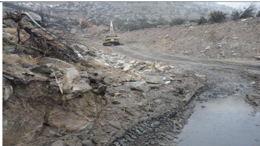
PHOTO 3 Upper South Culvert Addition
