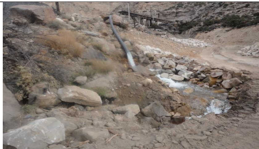
PHOTO 4 Extending the Disturb Area
